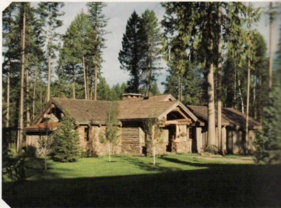
Preserving the towering 200-year-old tree in the front was a top priority for the Waggoners during construction of their guest cabin.
